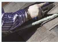
Roof Shingles & Siding
