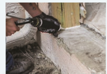
Plaster, Putties & Caulking
