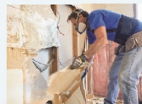
Drywall & Cement Sheets
